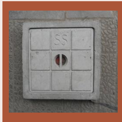
Manhole Cover RCC Mold
